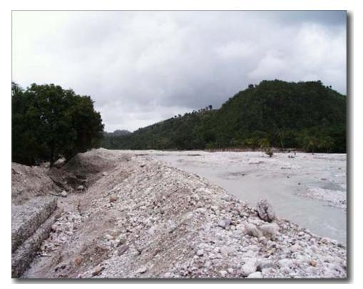
This photo, taken two weeks before the floods, shows the dyke construction (on the left) designed to keep the river within its banks. The main road is hidden to the extreme left (Photo courtesy Franco Gattigo, AECP)
